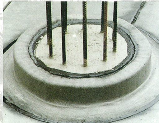
Detail at pile, using 20% SBS modified homogeneous bituminous membrane.
